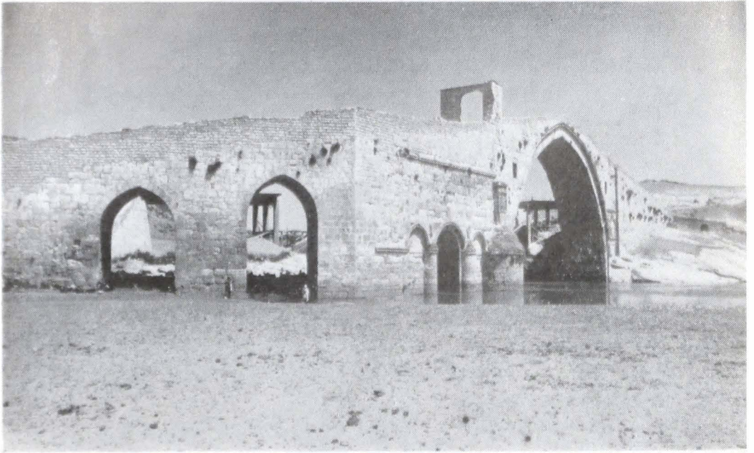
ABASSID BRIDGE E. OF SILVAN ON BATMAN SU: 1147 A.D.
